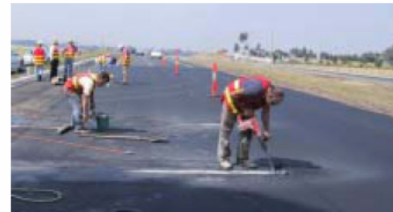
The sensors are installed in slots cut into the road surface (asphalt or concrete) which are grouted with a compound of epoxy and silica sand.
