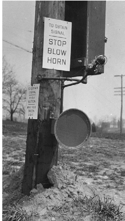
"To Obtain Signal - Stop Blow Horn," traffic-actuated signal light, Charles Adler, Jr. Collection, ca. 1920-1980
